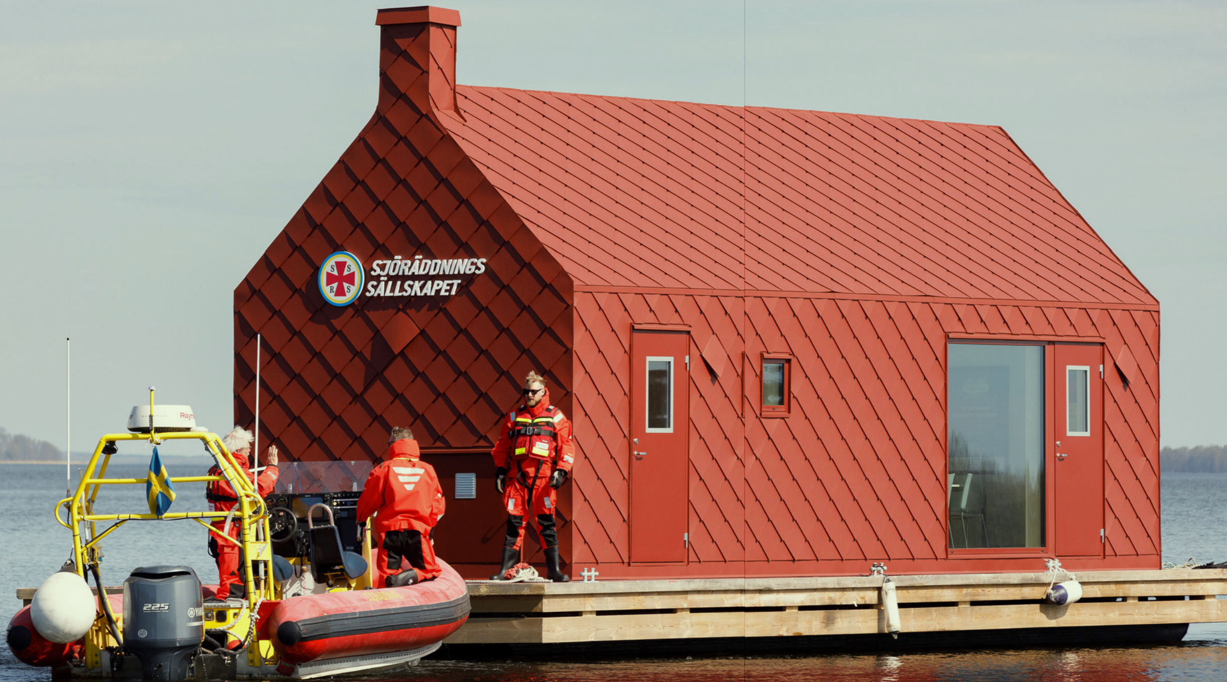
The Swedish Sea Rescue Society RS Hjälmarén base is on a former houseboat that has been converted into a floating station made of sheet metal. The building was one of six finalists in Plåtpriset 2022, an award celebrating innovative, sustainable buildings that use sheet metal facades.
