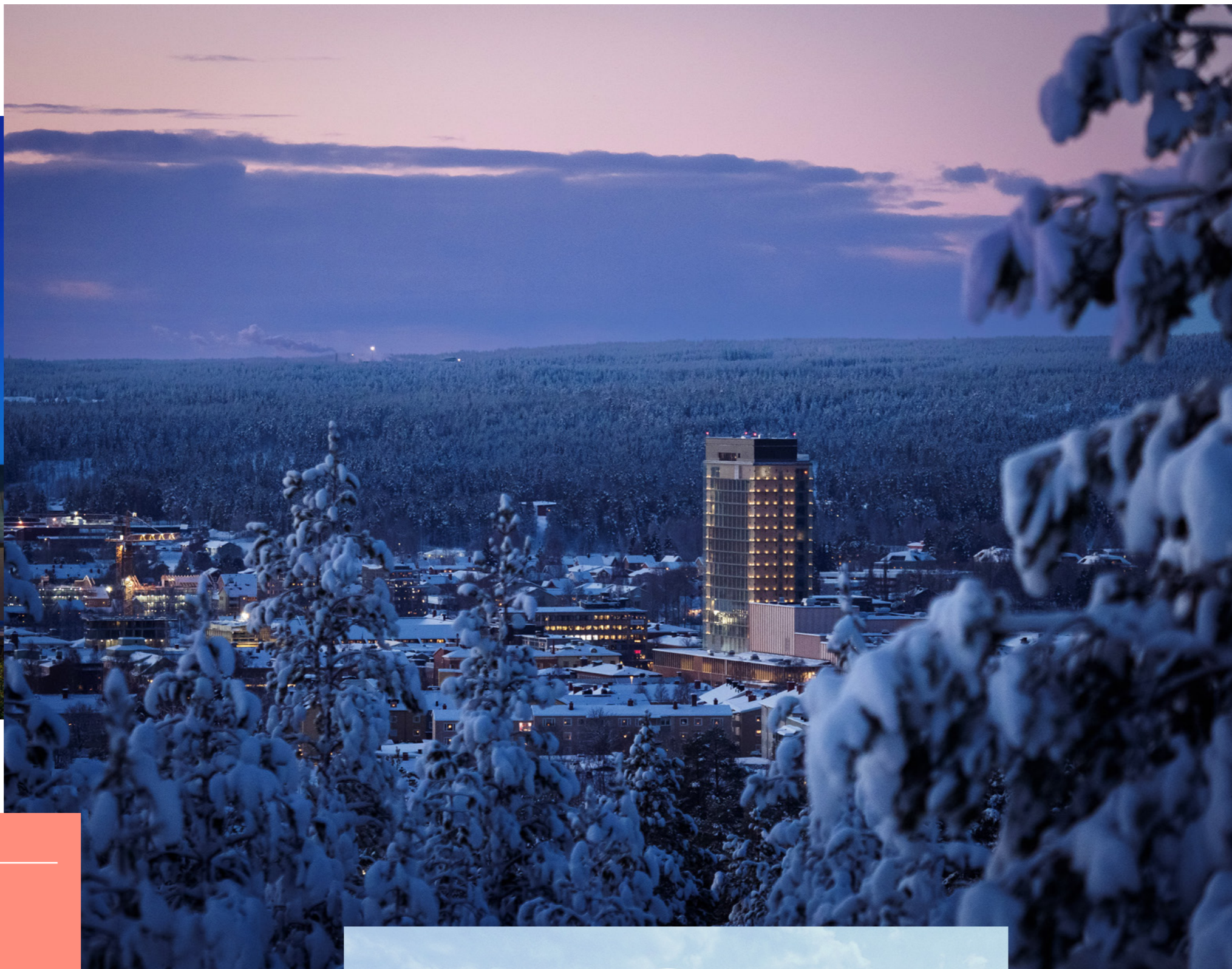
Sara Cultural Centre, Skellefteå. Winner of Global Vision Awards Travel + Leisure's 2022, International Award for Wood Architecture and WAF, Completed Buildings – Culture.
