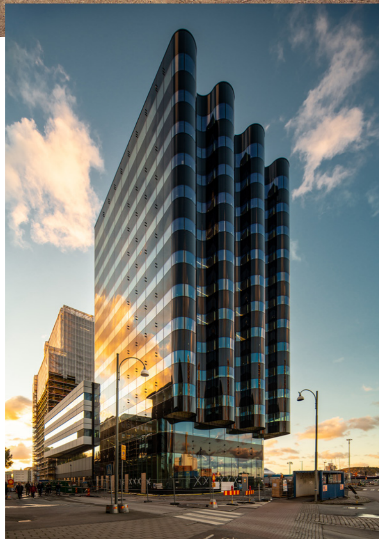
Våghuset office building, Gothenburg. Winner of Glaspriset glass prize.
