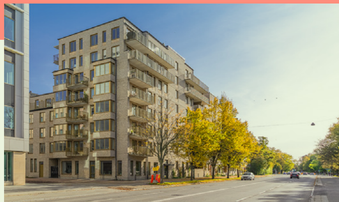
The tenant-owner housing blocks Operan and Operetten in Malmö provide housing for seniors in the heart of the city. The garden is an intimate, cosy place to socialise and the greenhouse is a place for gardening and celebrations.
