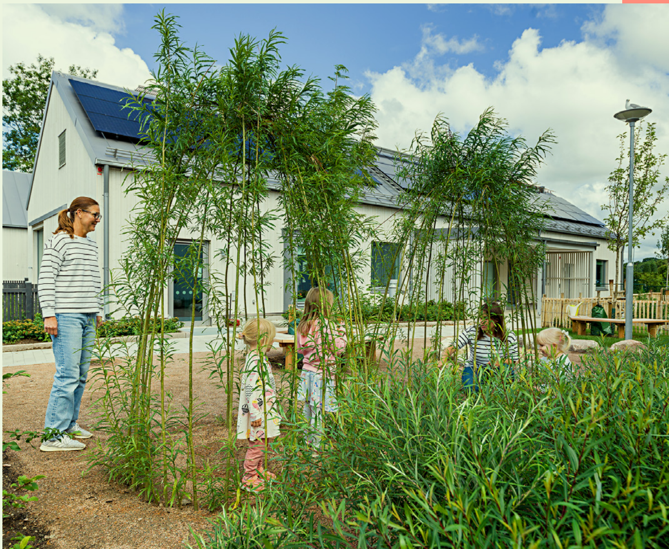
Vårhem preschool and parish hall creates a natural meeting-point between the children's and adults' world. The building signals closeness and a sense of small scale, and houses a preschool with two departments for 40 children in total and a parish hall with room for 50 people.
