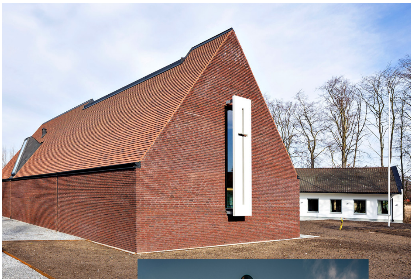
Torn Parish Hall, Lund. Winner of Facade of the Year 2022, new production.
